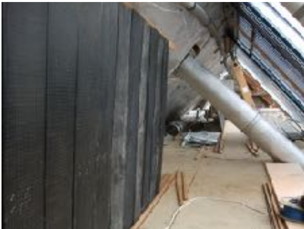
Fig.1. Converted stables loft. Polycarbonate roof to the right; thin black aluminium heat absorbing panels, left; chimney from supplementary wood boiler (on ground floor) in centre; behind the chimney at far end of loft, cardboard duct with two 7W 12V fans blowing warmed air into lounge below. Conventional vacuum domestic hot water tubes are visible top right.
