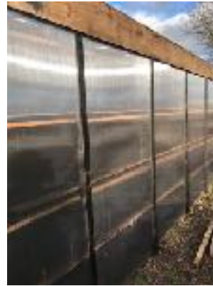
Fig.3 Kiln front with polycarbonate fitted
